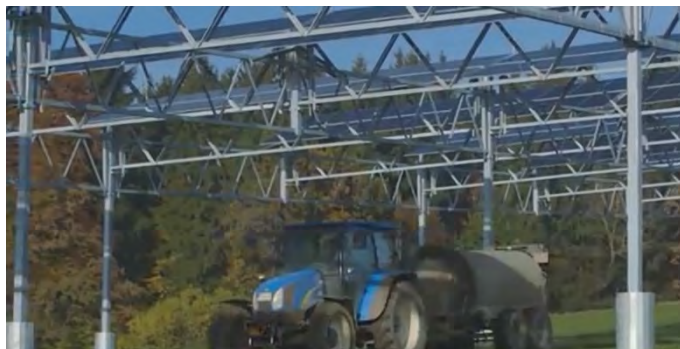
Figure 32: Example Agrivoltaic Installation
